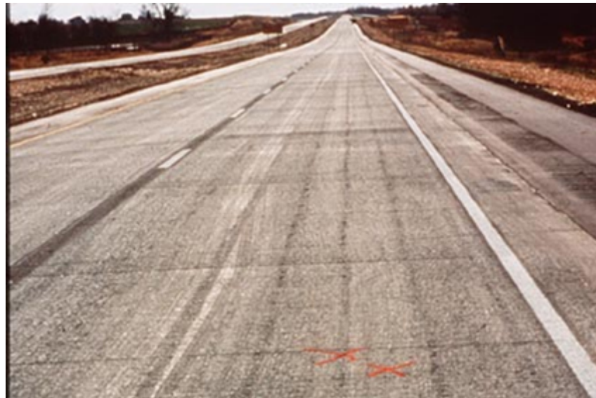
Figure 1.3 Longitudinal vibrator trails [4]
